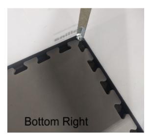
Tiles all with 24 3%" height and width will need the entire height of every tooth along two perpendicular sides removed. They will also need part (if not all) of the height of all teeth along the remaining two edges removed.
